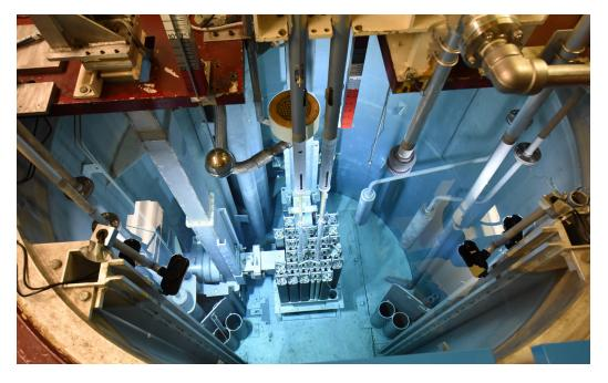
The NRAD reactor provides a neutron source for indirectfilm and digital radiography of irradiated fuels and materials, neutron computed tomography and neutron diffraction
